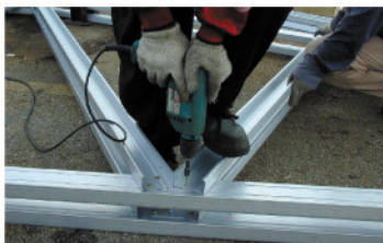
Step 4 : Easy and quick to install by using self drilling screw
