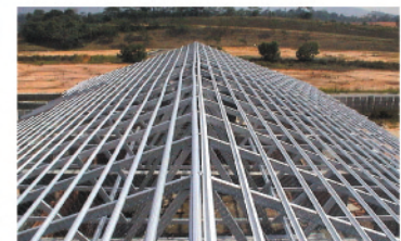
Step 6 : Roof truss system. No painting, cutting or welding at site
