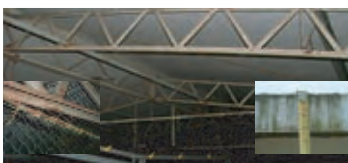
High Corrosivity, Fungi & Lichien inside panel
