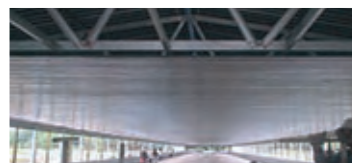
Add-on metal ceiling for optimize ventilation
