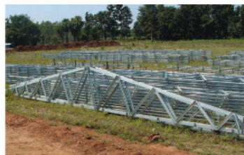
Step 5 : Light Weight trusses are ready to install
